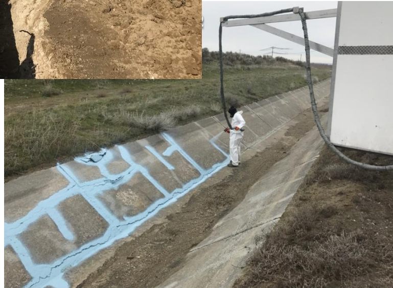
Crack Sealing
