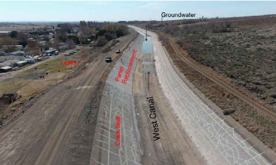
West Canal in South Ephrata where repairs are needed.
